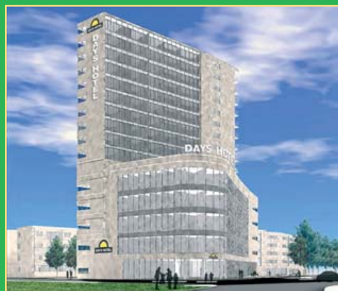
Days Hotel in Santry Cross is expected to open on 15th May, as part of the regeneration project
